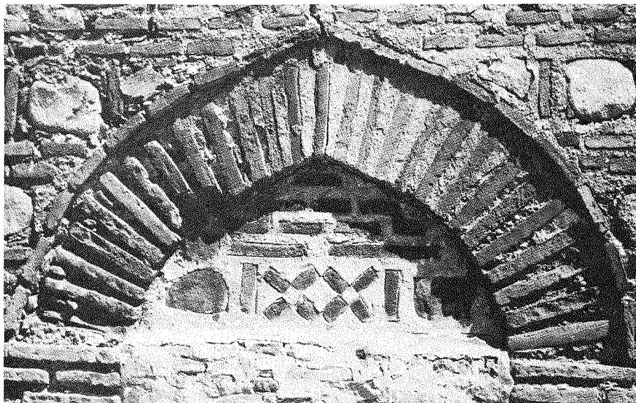
Fig. 1. Example of ornamental brickwork. Fethiye Cami 1430/35, Kustendil, West Bulgaria.
